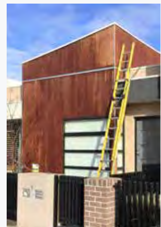
CLEANING: Wash the boards with a product like Intergrain Reviver or Cabots Deck Clean and a firm brush.
