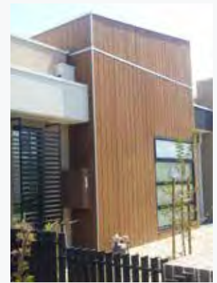
4 MONTHS: The board shows signs of lightening.
